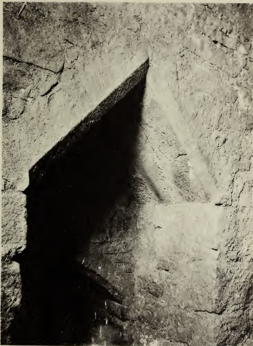
(FIG. 10) VIEW OF INNER SIDE OF MAIN ENTRANCE TO TOWER, SHOWING LATER ADDITION TO THICKNESS OF WALL
